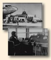
Cleveland's airport opened the first radio-equipped control room in 1930. Soon, nearly all airlines were equipping aircraft for radio navigation. By 1932, the Commerce Department had installed 83 radio beacons across the country. These transmitted directional beams that pilots could follow to their destinations.
